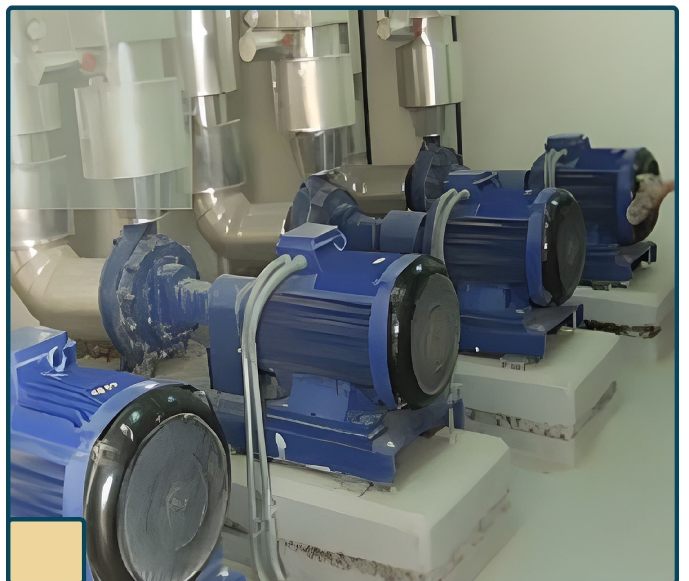
Centrifugal pump (End suction pump )
